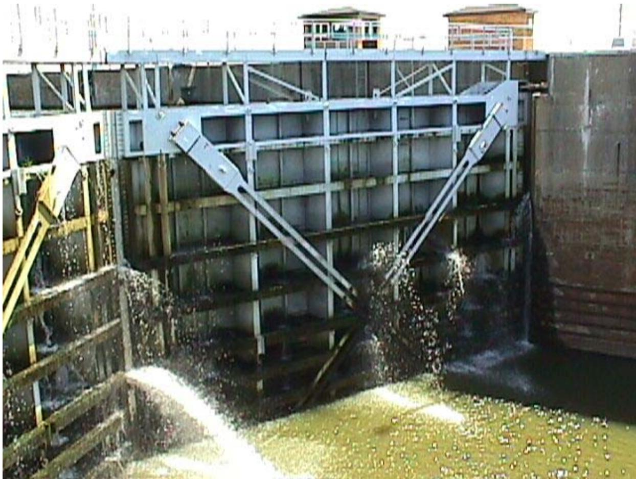
Leaking Spare Miter Gates, Lock and Dam 19, Mississippi River
