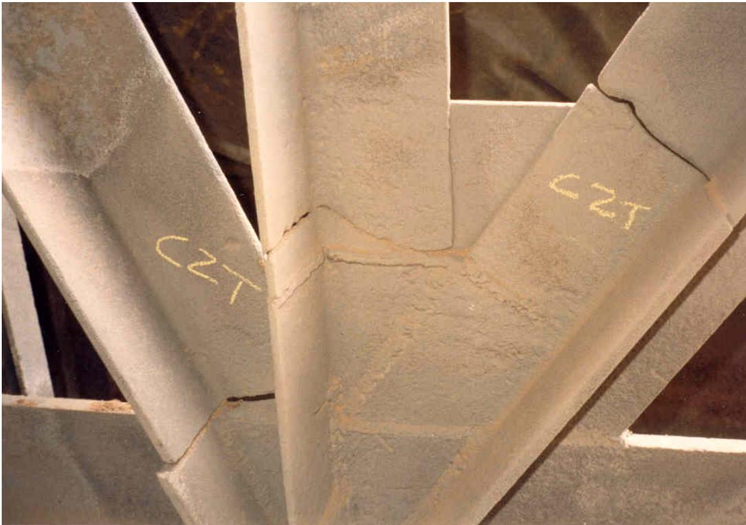
Lock 27: Serious fatigue damage to original main chamber upstream lift gate leaf.
