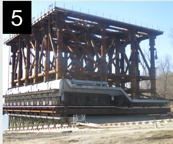
1. Upper Pier Build-out (Nos. 1-6) 2. Dredging Boat Harbor 3. Deploying Diver 4. TG-1 resting on dogging beams 5. NP-2 moving down skidway 6. NP-2 Tremie Placement
