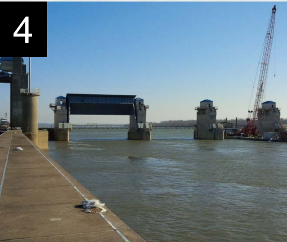
1. Upper Pier Build-out (Nos. 1-6) 2. Dredging Boat Harbor 3. Deploying Diver 4. TG-1 resting on dogging beams 5. NP-2 moving down skidway 6. NP-2 Tremie Placement
