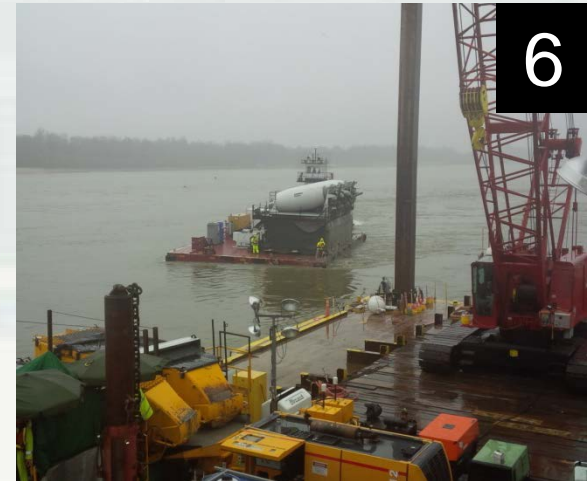
1. Upper Pier Build-out (Nos. 1-6) 2. Dredging Boat Harbor 3. Deploying Diver 4. TG-1 resting on dogging beams 5. NP-2 moving down skidway 6. NP-2 Tremie Placement
