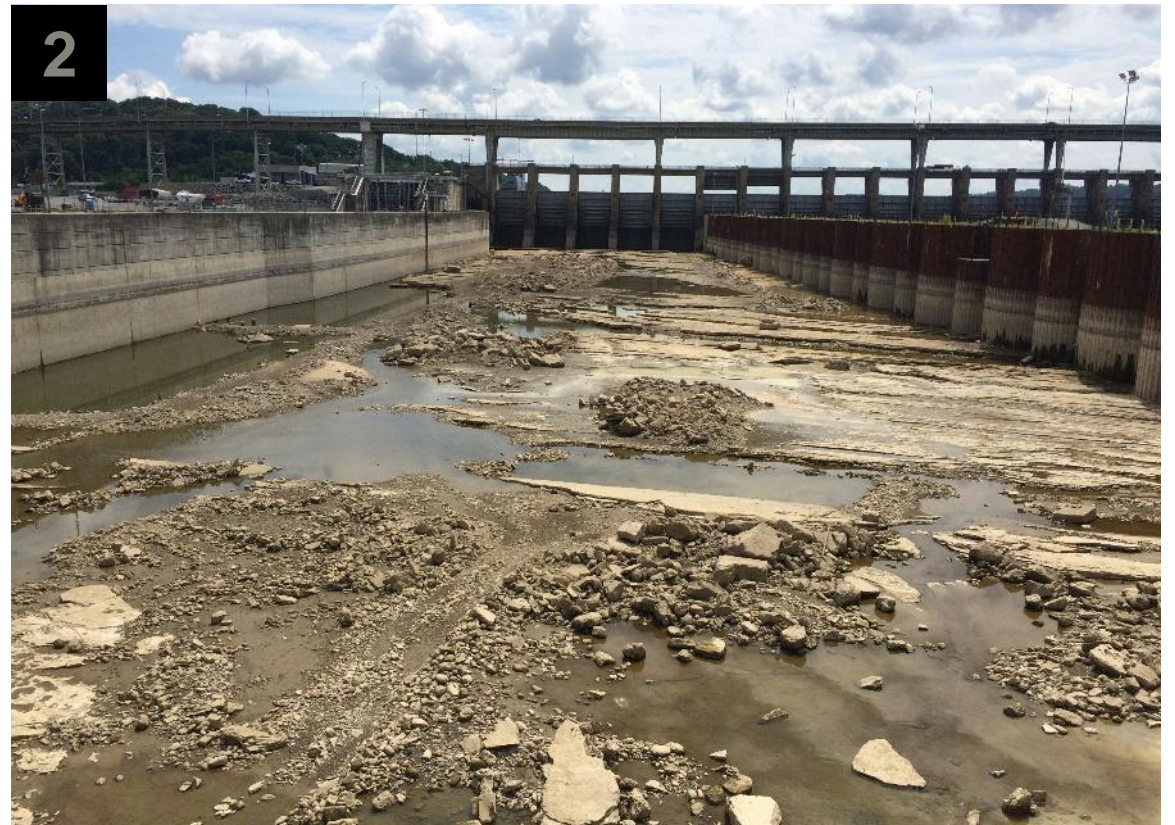
1. Cofferdam completed in 2012; 2. Cofferdam dewatered looking Upstream in June 2016 during Cofferdam Stabilization contract
