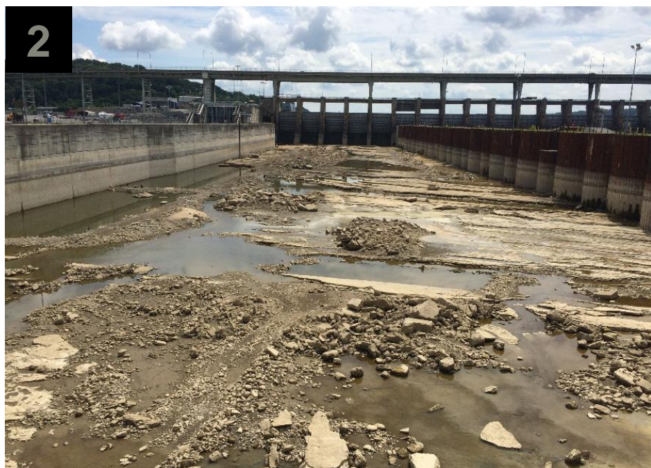
1. Cofferdam completed in 2012; 2. Cofferdam dewatered looking Upstream in June 2016 during Cofferdam Stabilization contract; 3. Site visit by LRD Commander, BG Mark Toy, Congressional Staffers, and Navigation Representatives on 25 January 2017.
