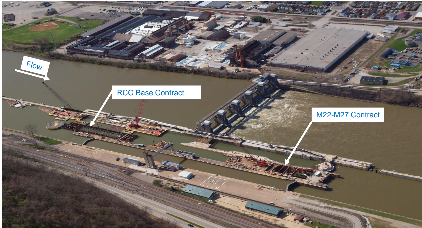
Aerial view of Charleroi Lock Construction
