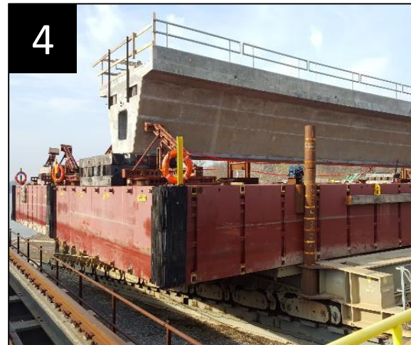
4 Service Bridge (SB) No. 5
