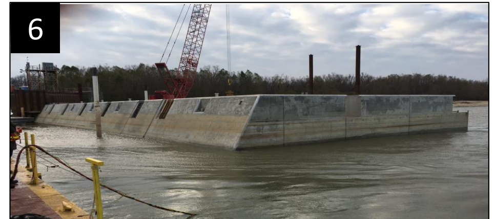
Left Boat Abutment
