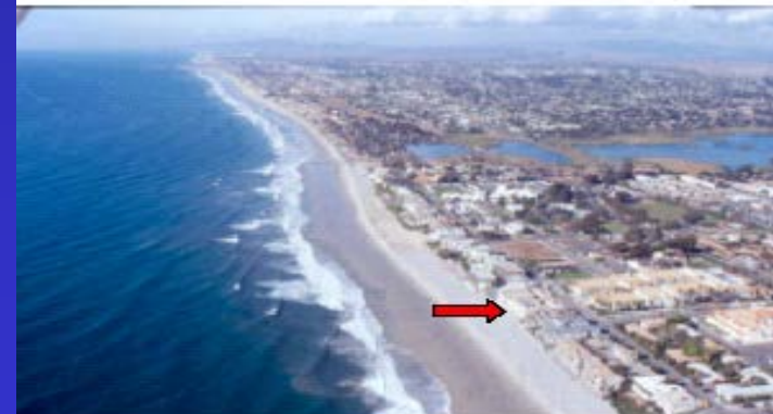
Plate 5.10 Post-nourishment condition at North Carlsbad site, November 2001 (arrows point to approximately the same location on each photo)
