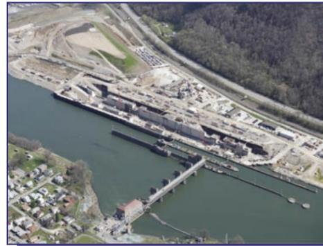
The 1200-foot locks can accommodate a tow of 17 barges plus the towboat, while the 600-foot locks can accommodate at most eight barges plus the towboat. The lock size and tow size are critical factors in the amount of cargo that can pass through a lock in a given period of time. Since many of today's tows operate with 12 or more barges, passing through a 600-foot lock requires the tow to be “cut” into two sections to pass the lock. Such multiple cuts can be
