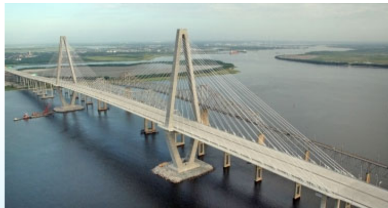
Cooper River Bridge
