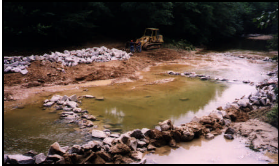
Bendway Weirs with longitudinal peaked stone toe protection Figure 34 Ft. Belvoir, Va.
