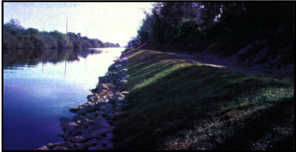
Riprap at Toe of Streambank with Vegetation Figure 26b
