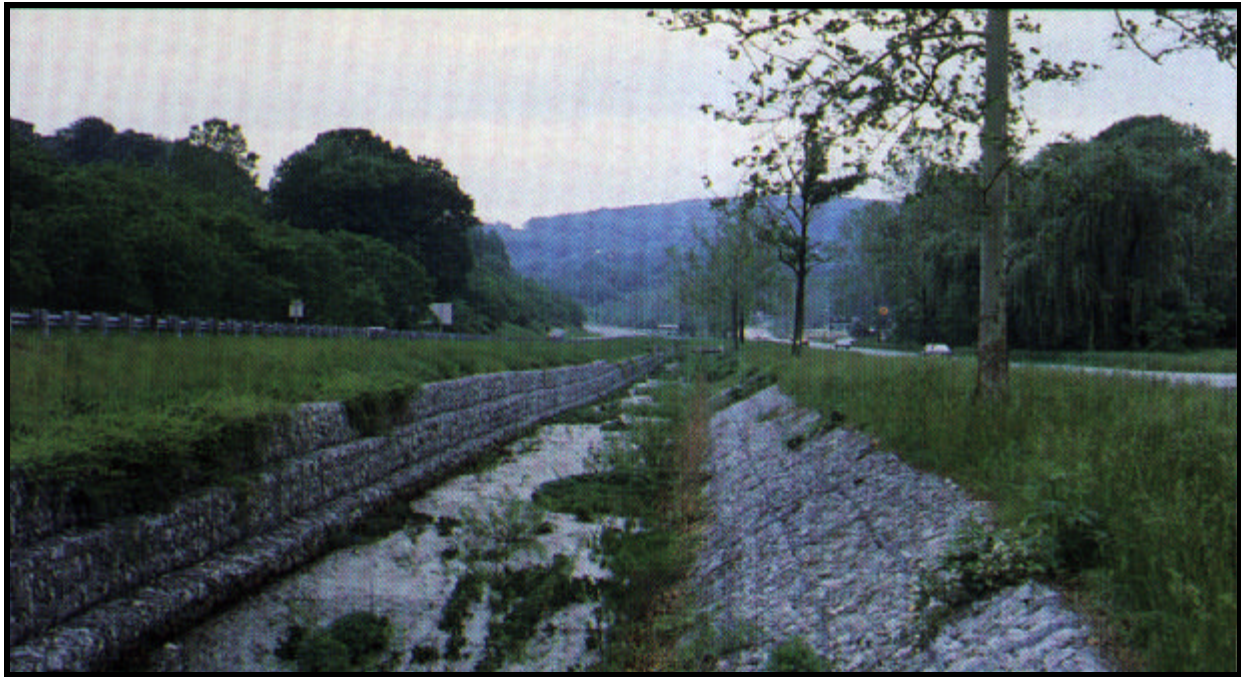
Gabions (left bank) and Gabion (Reno) Mattress (right bank) photo courtesy of "Maccaferri Gabions, Inc."
