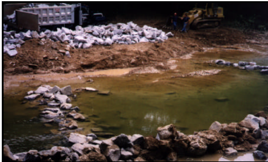
Bendway Weirs with longitudinal peaked stone toe protection Figure 34a
