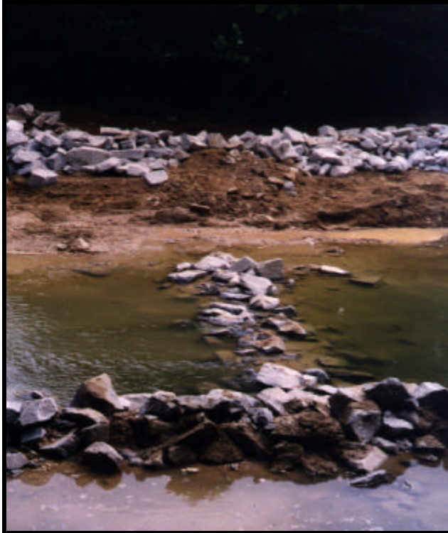
Closeup of Bendway Weir Ft. Belvoir, Va.
