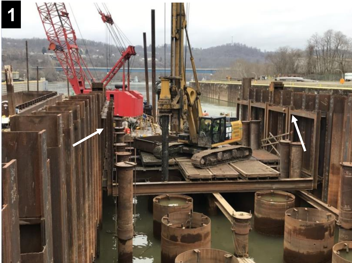
1 –M22-M27 Contract, M27 Drilled Shaft Construction 2 –RCC Contract, Base, Cofferdam Planned Flooding
