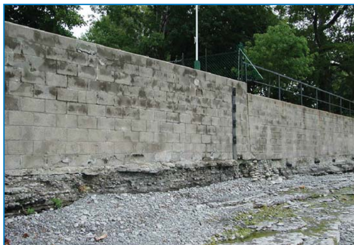
Figure C-3: Example of existing shore protection at risk of undercutting during low water periods
