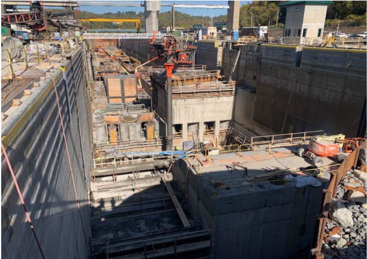
Monongahela River Charleroi Lock Construction
