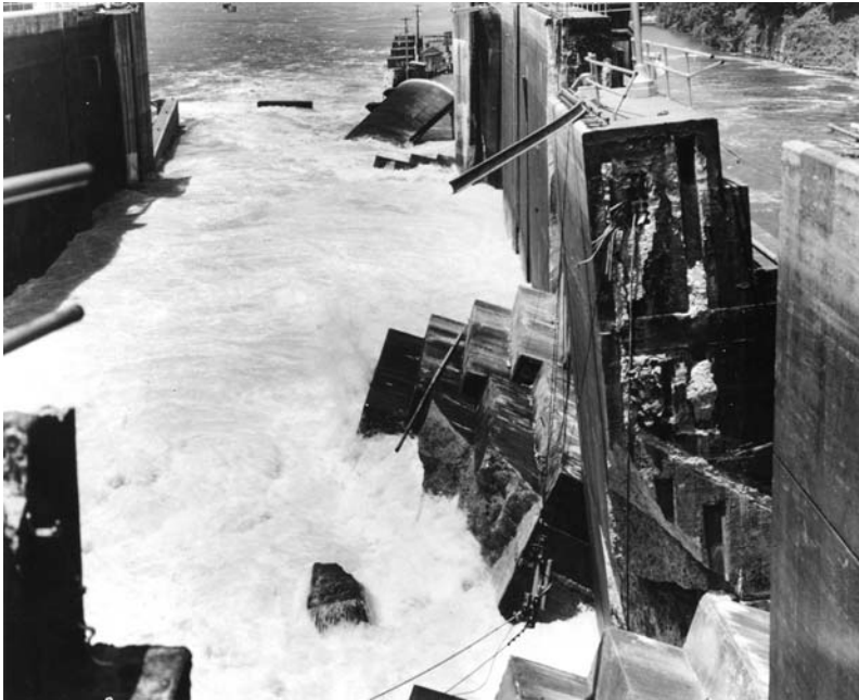
Collapse of Wheeler Lock on the Tennessee River, 1961.
