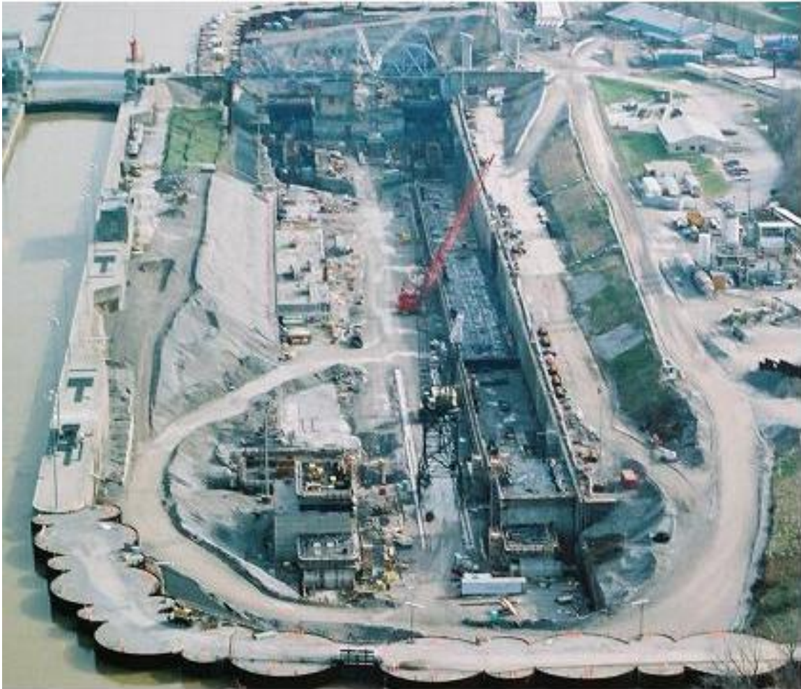
Ongoing Construction at the McAlpine Locks and Dam, Ohio River, January 2005
