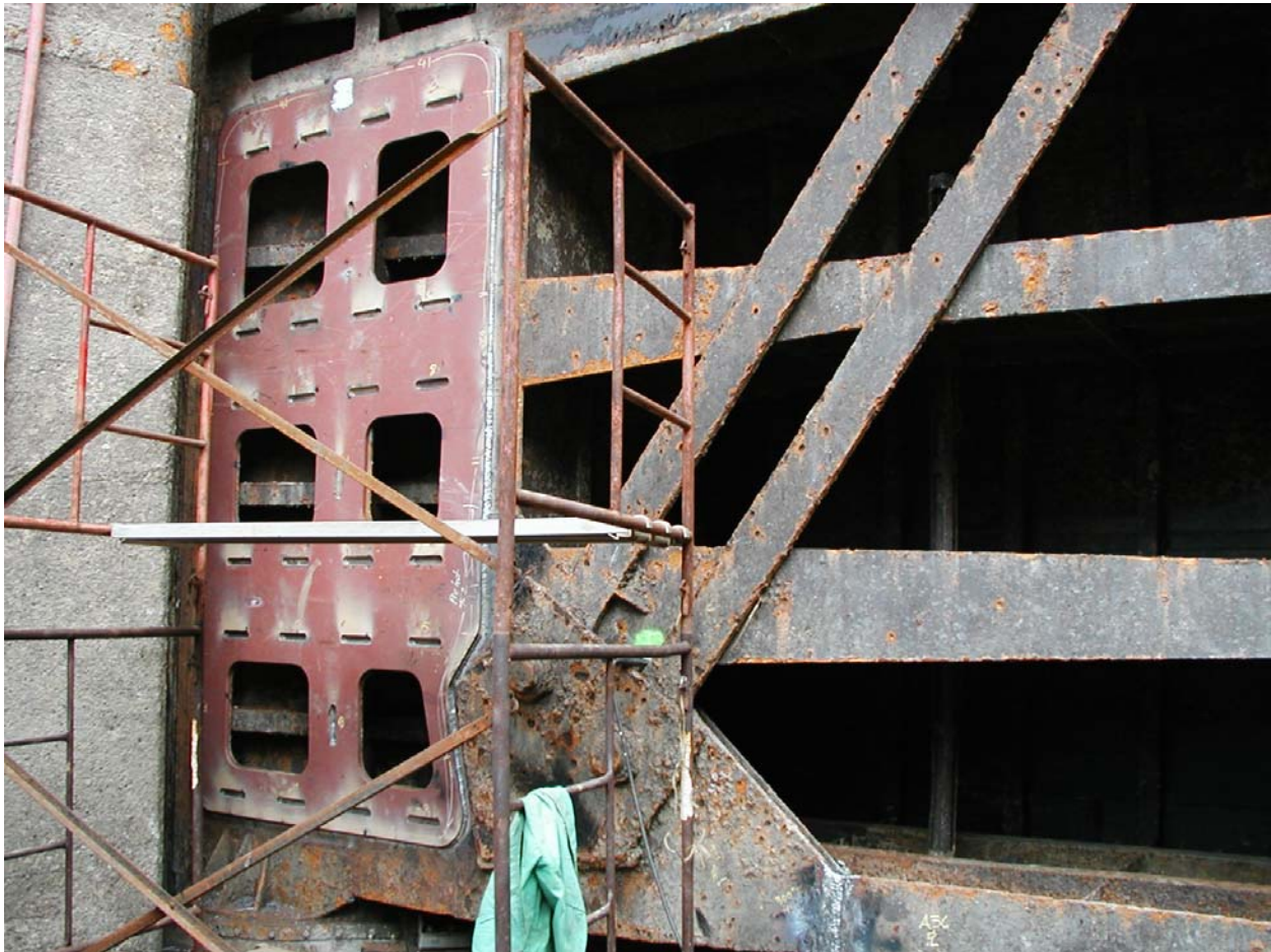
Emergency Gate Repair at McAlpine Lock on the Ohio River, 2004.
