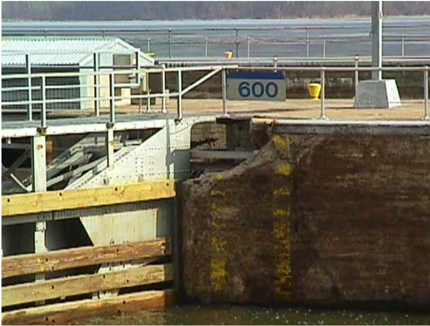
Miter Gate Concrete at Lock and Dam 11, Mississippi River
