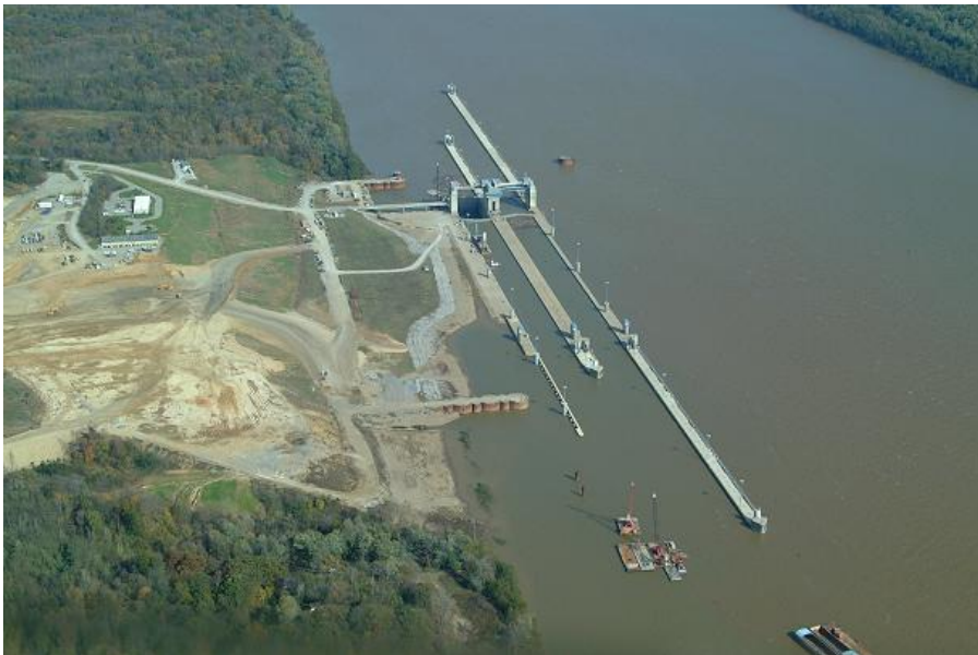
Olmsted Locks and Dam Construction Progress, November 2004
