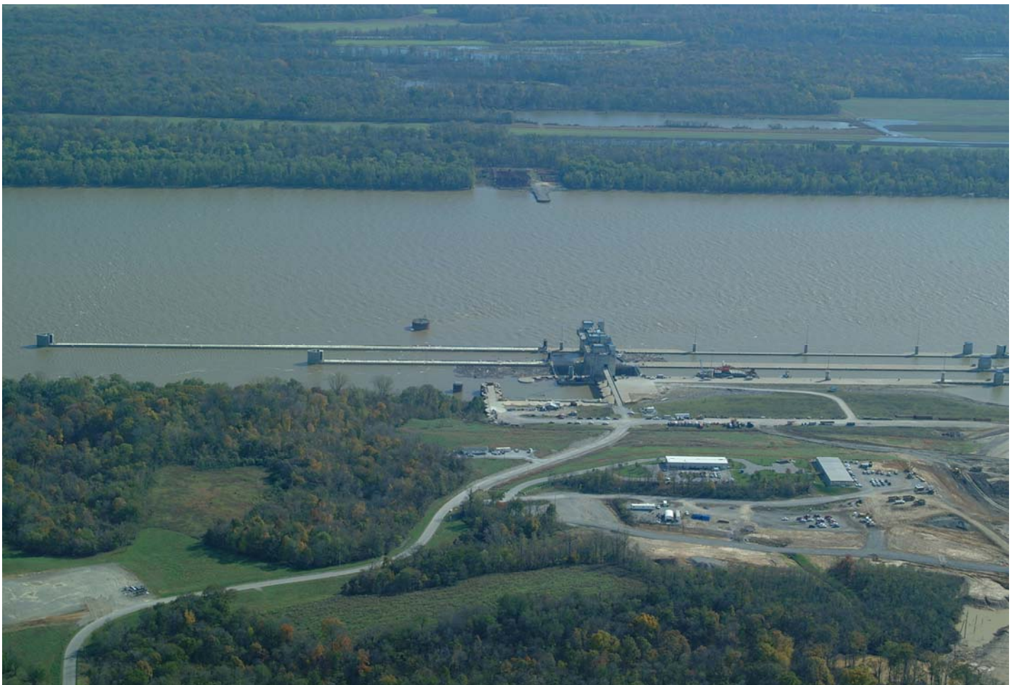
Olmsted Project: New Locks Await Construction of Dam
