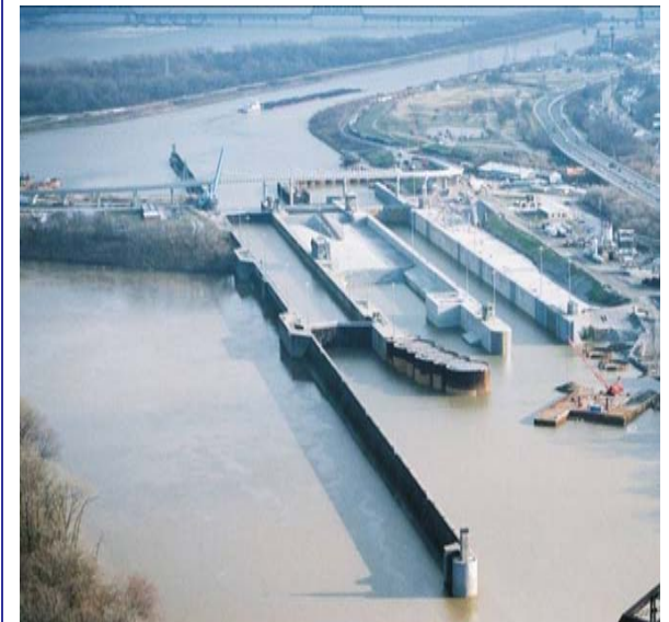
McAlpine Locks and Dam Project, Ohio River Construction of New Lock.
