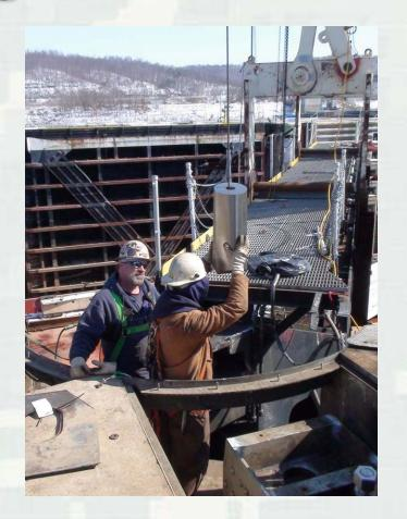
Replacing anchorage arms, links and pins
