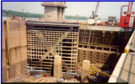
Failing Lock Gates
