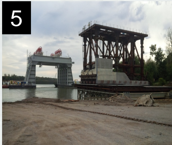
1. Aerial Photo - August 2014 2. TG-1 transiting L&D 52 3. Testing NP-1 Wicket Gates 4. Setting bulkheads Bay No. 1 5. RBA moving down skidway 6. Setting RBA/Erecting TG-1
