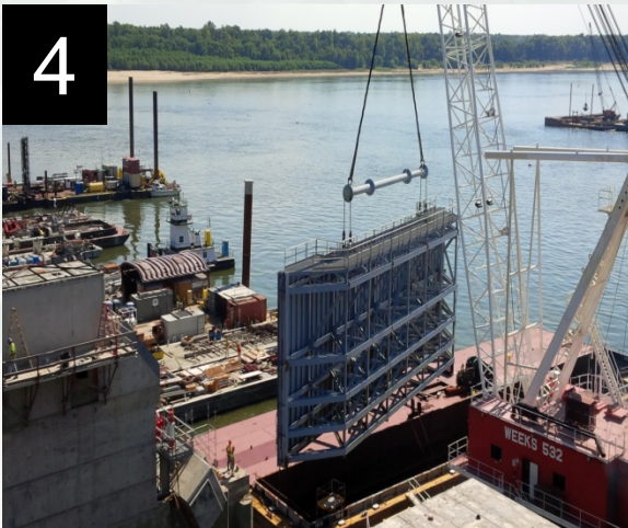
1. Aerial Photo - August 2014 2. TG-1 transiting L&D 52 3. Testing NP-1 Wicket Gates 4. Setting bulkheads Bay No. 1 5. RBA moving down skidway 6. Setting RBA/Erecting TG-1
