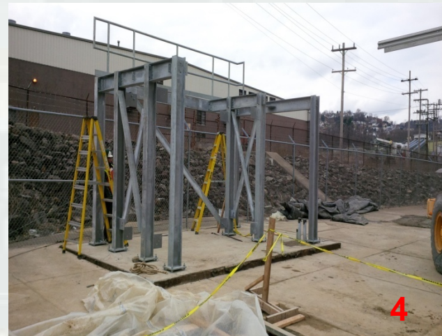
Emptying Basin Contract: 1 - Pre-Cast Basin Units; 2 - Foundation Drilled Shafts . M22-M27 Contract: 3 - Emergency Generator Pad Reinforcement; 4 - Emergency Generator Platform
