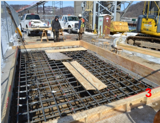
Emptying Basin Contract: 1 - Pre-Cast Basin Units; 2 - Foundation Drilled Shafts . M22-M27 Contract: 3 - Emergency Generator Pad Reinforcement; 4 - Emergency Generator Platform
