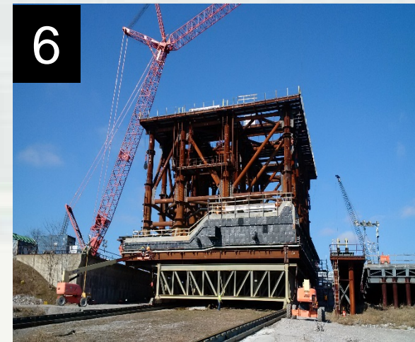
1. First Commercial Lockage 2. River Chamber Unwatering 3. NP-3 Wicket Installation 4. TG-1 Cylinder Installation 5. TG Bay 1 Unwatering 6. NP-6 Transiting Skid Way
