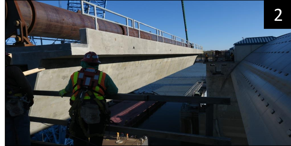
2 Installation of Service Bridge Nos. 3 & 4
