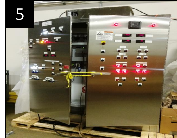
5 TG Control Cabinet
