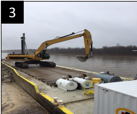
3 River Dike No. 4
