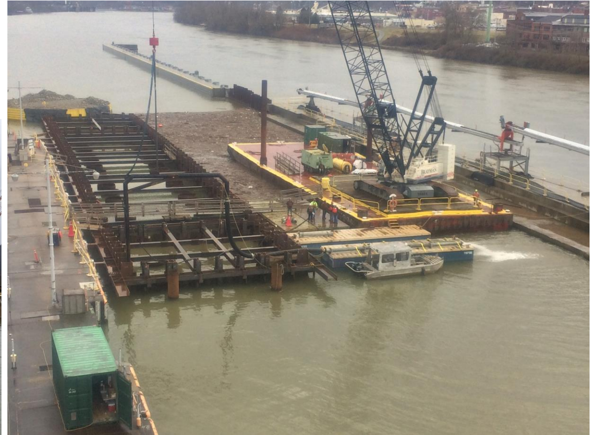
RCC Contract – Excavation by airlifting inside bellies of coffer box sheet piling
