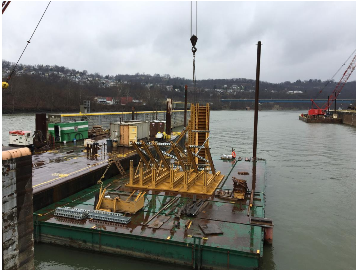
M22-M27 Contract – Cofferdwall Formwork
