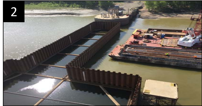
Left Boat Abutment (LBA) Cofferdam
