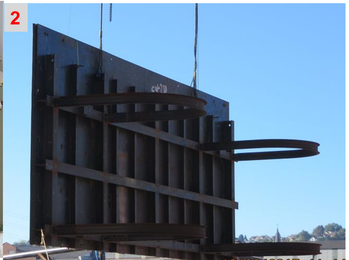
1 - River Chamber Completion Contract & M22-M27 Contract aerial View 2 - RCC Base Contract: M2/M3 Tremie Partition
