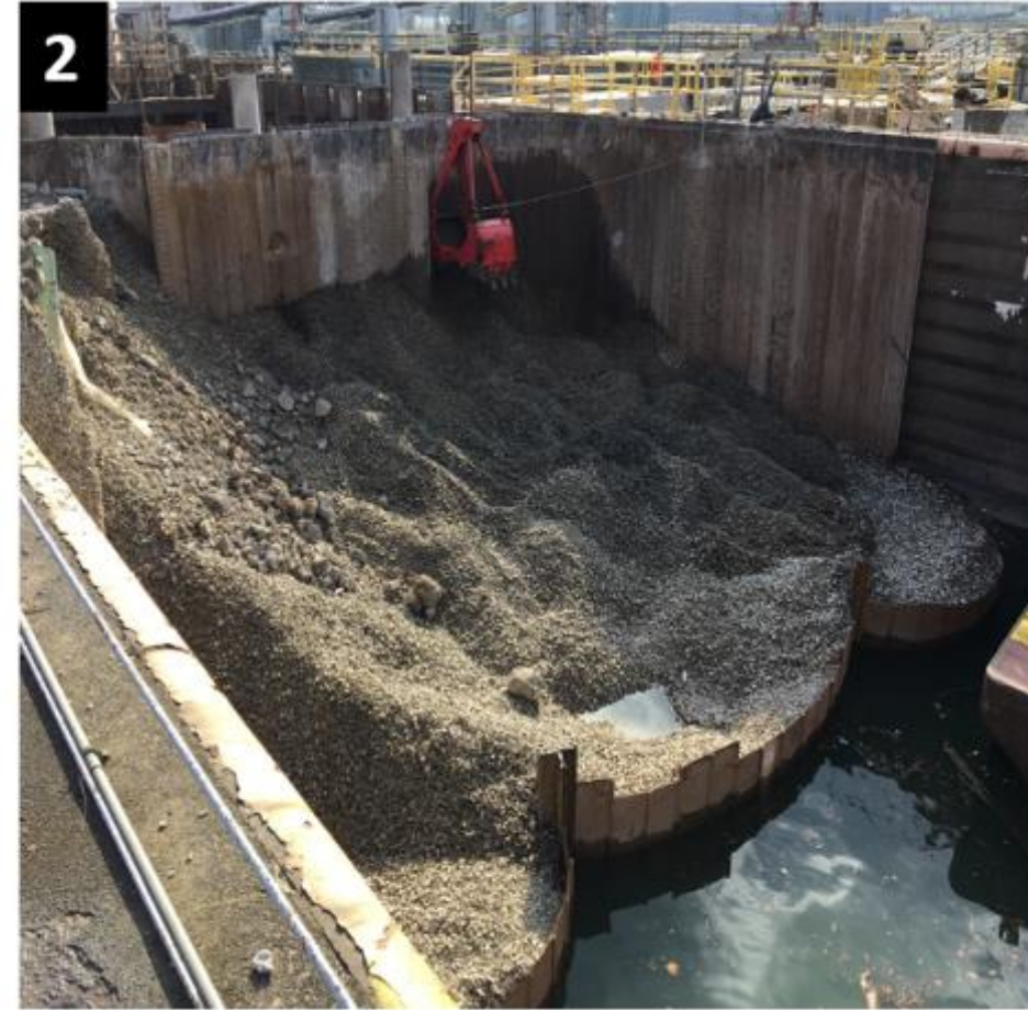
1 - River Chamber Completion Contract Dewatered M2-M6 Coffebox 2 - M22-M27 Contract Removal of the D/S Closure Cell
