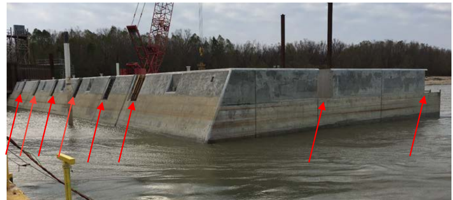
Left Boat Abutment – Final Concrete Placement
