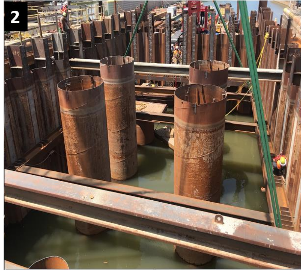
1 - River Chamber Completion Contract Dewatered M2-M6 Cofferdbox 2 - M22-M27, Installation of Lower Water in M23/M24 Cofferdbox
