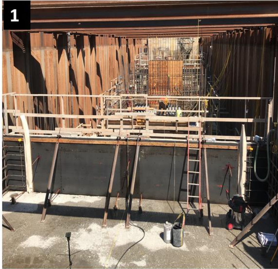
1 - River Chamber Completion Contract Dewatered M2-M6 Cofferdbox 2 - M22-M27, Installation of Lower Water in M23/M24 Cofferdbox
