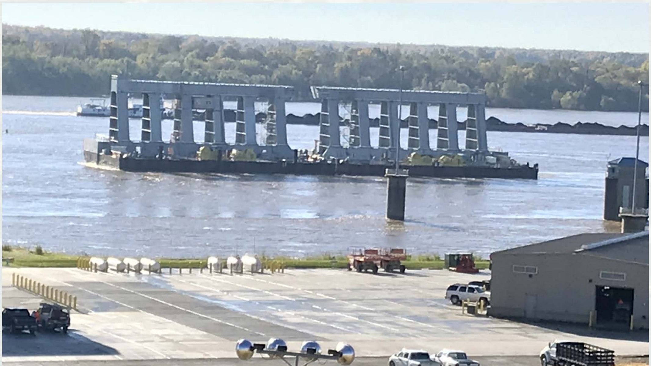
Worlds largest catamaran barge leaving the site.
