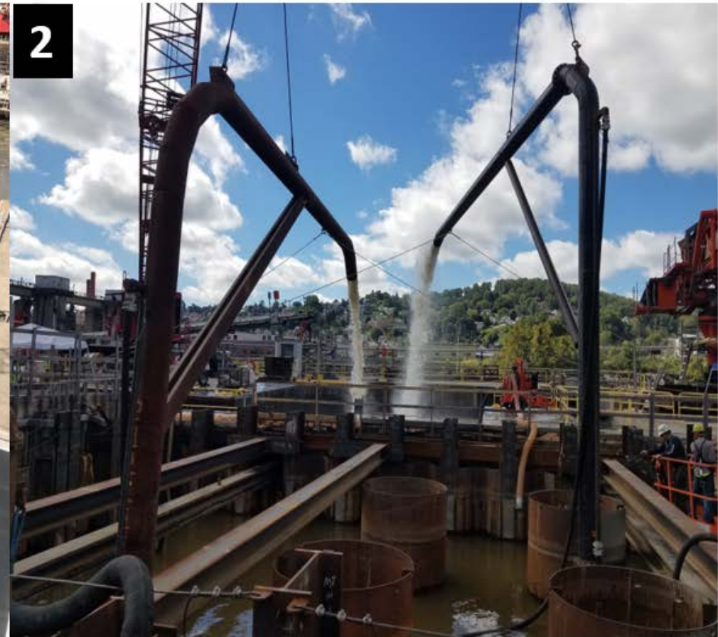
1 - River Chamber Completion Contract, M16 Cofferdbox after high water event first week of October 2 - M22-M27 Contract, Airlifting in Cofferdbox M23
