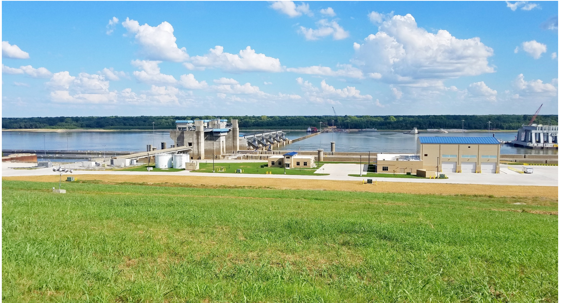
Olmsted Locks and Dam September 2018
