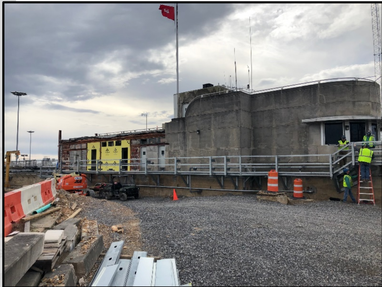
Operations Building modifications and catwalk
