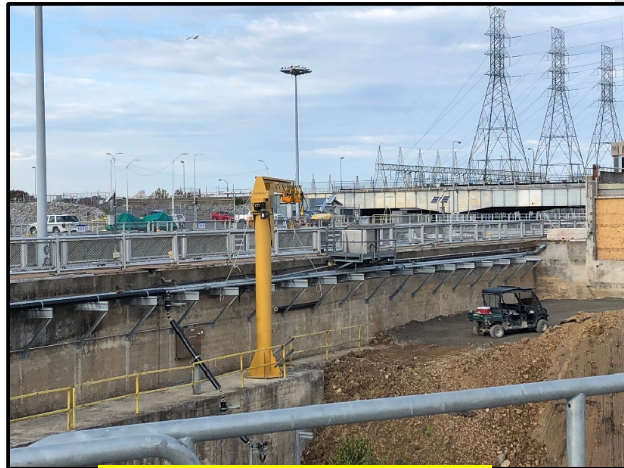
Utility brackets & jib crane on lock wall
