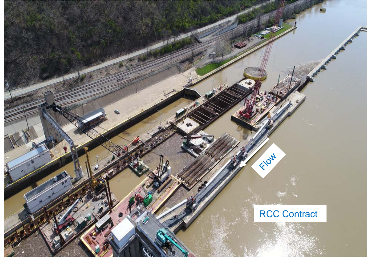
Aerial views of Concrete Batch Plant and Charleroi Lock Construction
