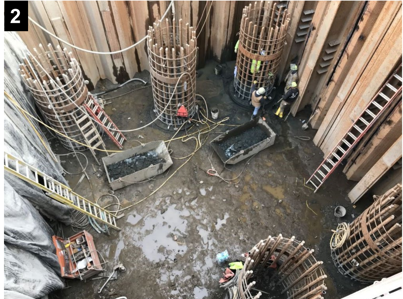
1 – Stilling Basin Contract , grout bag demonstration setup 2 – M22-M27 Contract, M25 tremie seal and drilled shafts
