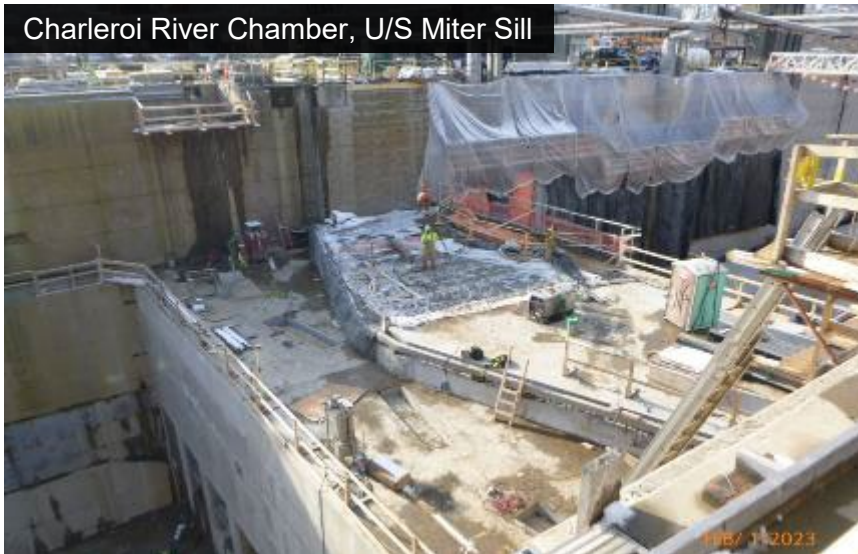
Charleroi River Chamber, looking downstream at U/S miter sill and lock filling ports
