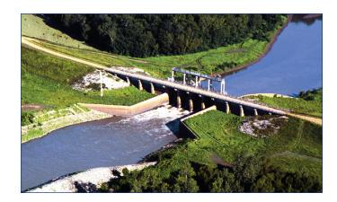
projects operate together as a system. During the low flow season, the storage projects release water to increase downstream flows, some or all of which are used to increase power generation at downstream run-of-river projects. Power generation is only one of the objectives of these storage
