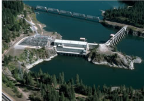
Figure 17. Photo of dam.
